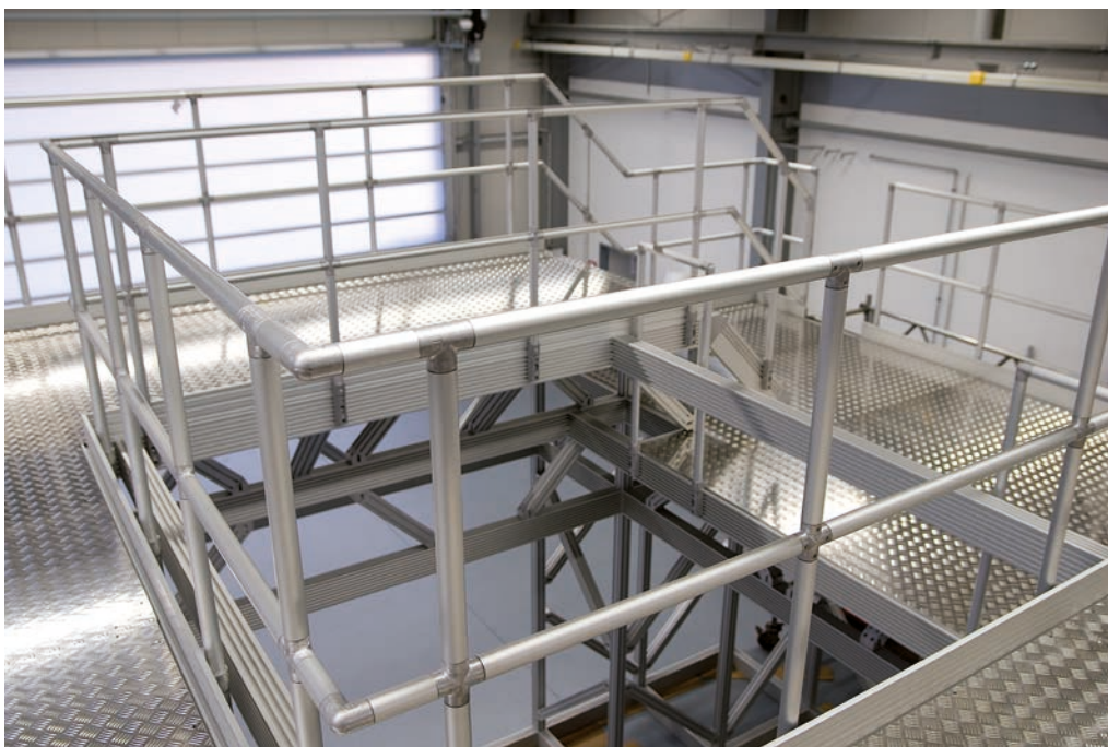
Working platform with ITAS railing
