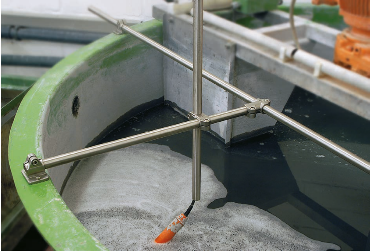
Simple probe fixation in an aggressive environment.
